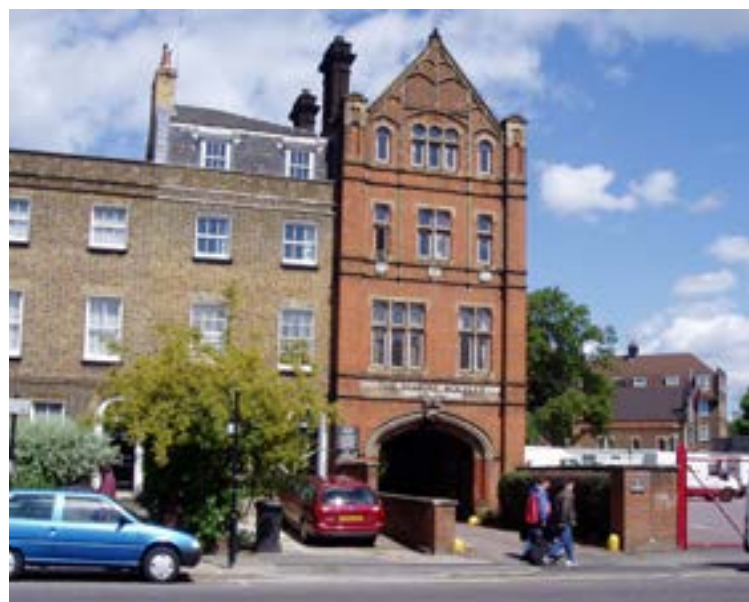
Entrance to IFSMA Office complex at 202 Lambeth Road.
