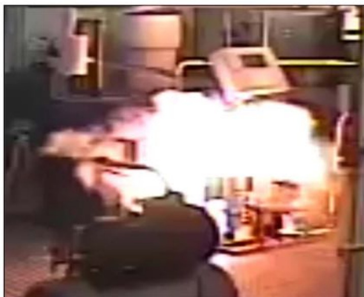
Figure 3: Engine room CCTV of ME2 engine fire
